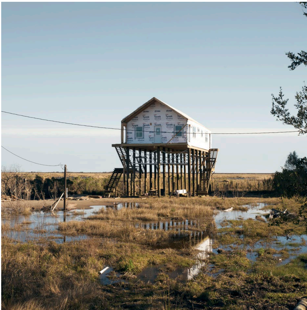
VIRGINIA HANUSIK, Construction near Lake St. Catherine, Orleans Parish, 2020.
