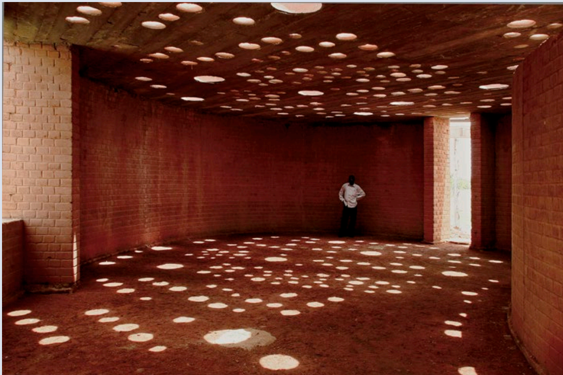
KÉRÉ ARCHITECTURE, Gando Primary School Library . Copyright Kéré Architecture.
