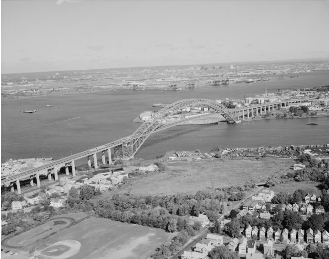
Bayonne Bridge, from over Staten Island looking north. Photo by John T. "Jet" Lowe, 1991. Courtesy the Library of Congress Prints and Photographs Division.
